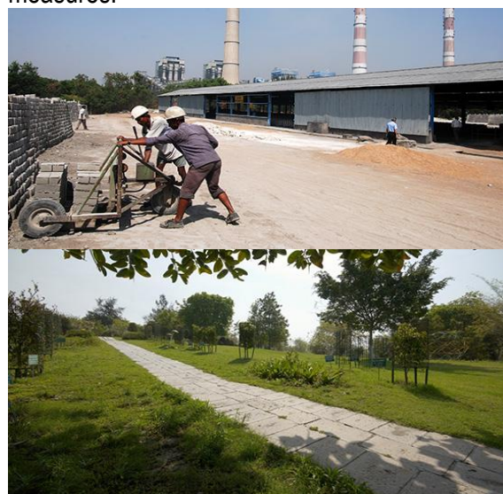
Figure 1: Paver blocks using Fly Ash at NTPC and its utilization within premises
