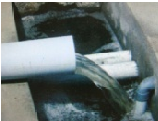
Figure 1. Contaminated water drainage
